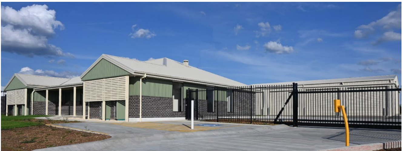
NEWA’s newly completed facility showing secure fencing, access control, CCTV and the depot in the rear.
